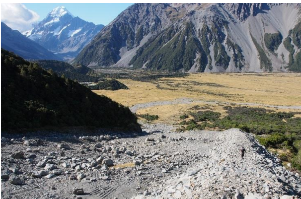
Figure 9: Completed diversion berm looking downslope.
