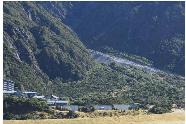
Figure 11: Completed diversion berm viewed from Aoraki Mt. Cook Village.
