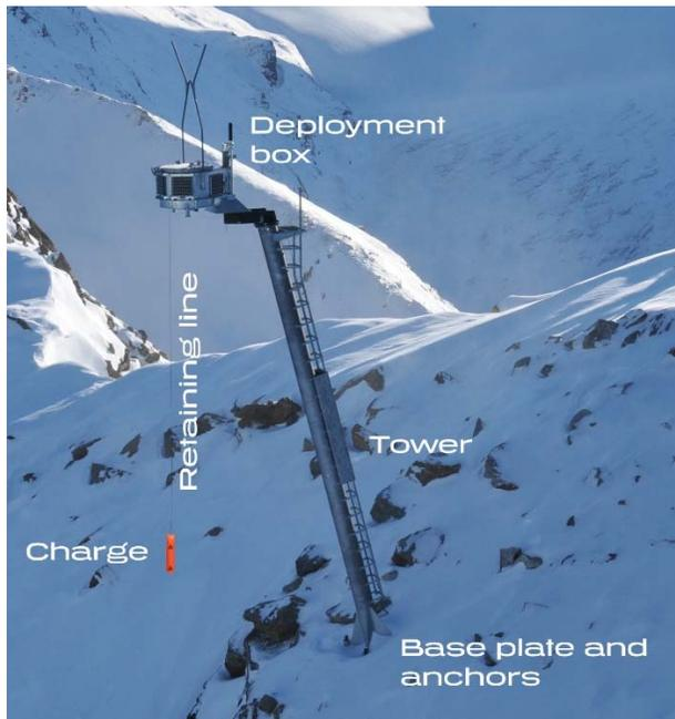
Figure 2. System description of RACS tower used in 3VG.
